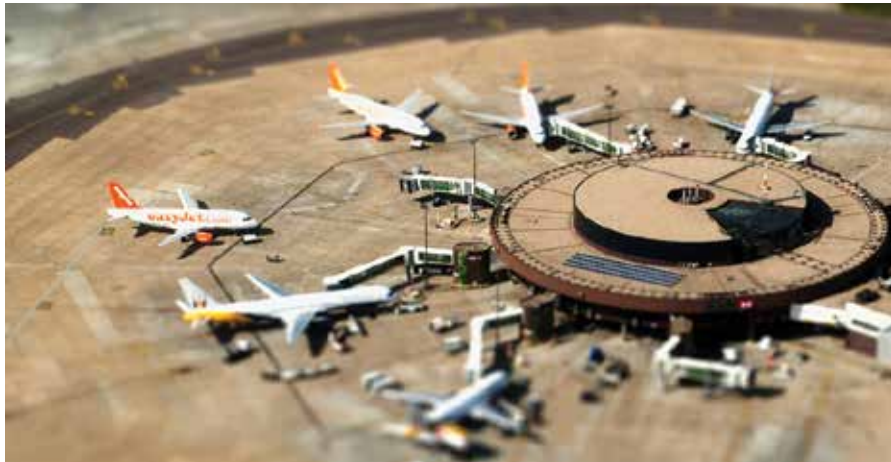
Gatwick airport by Stav via flickr
