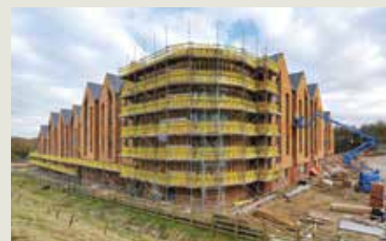
Chamberlain Manor Construction, Pentland
